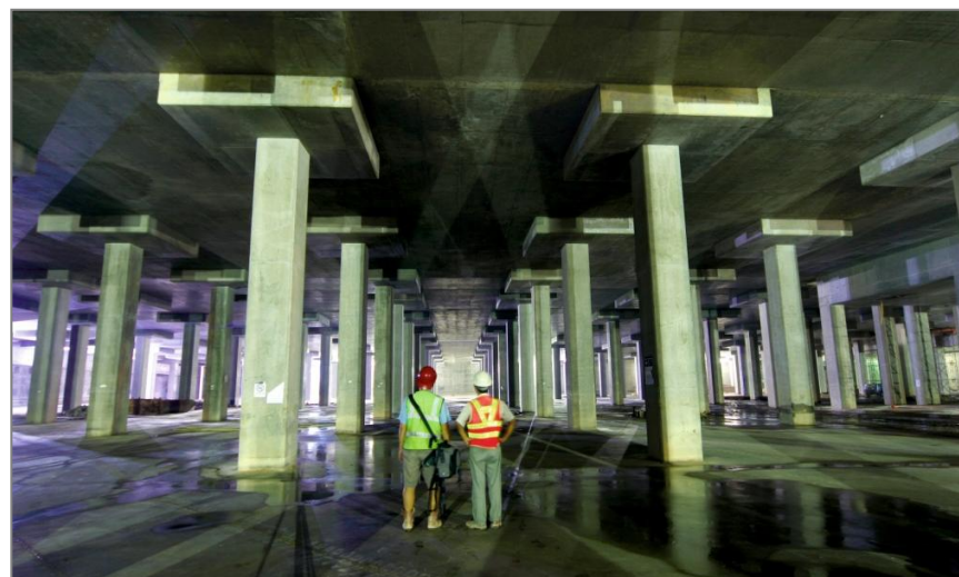
Figure 42 Tai Hang Tung Underground Stormwater Storage Scheme
