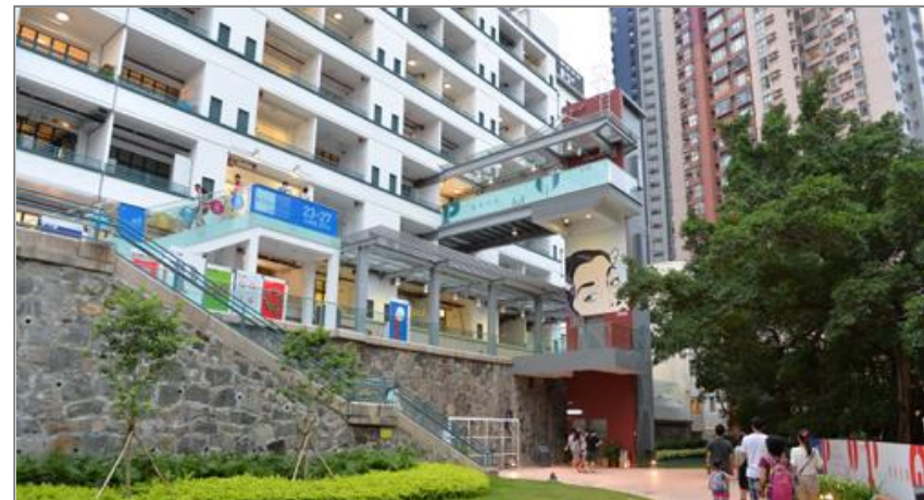
Figure 46 PMQ - Creative Industries in Historic Building
